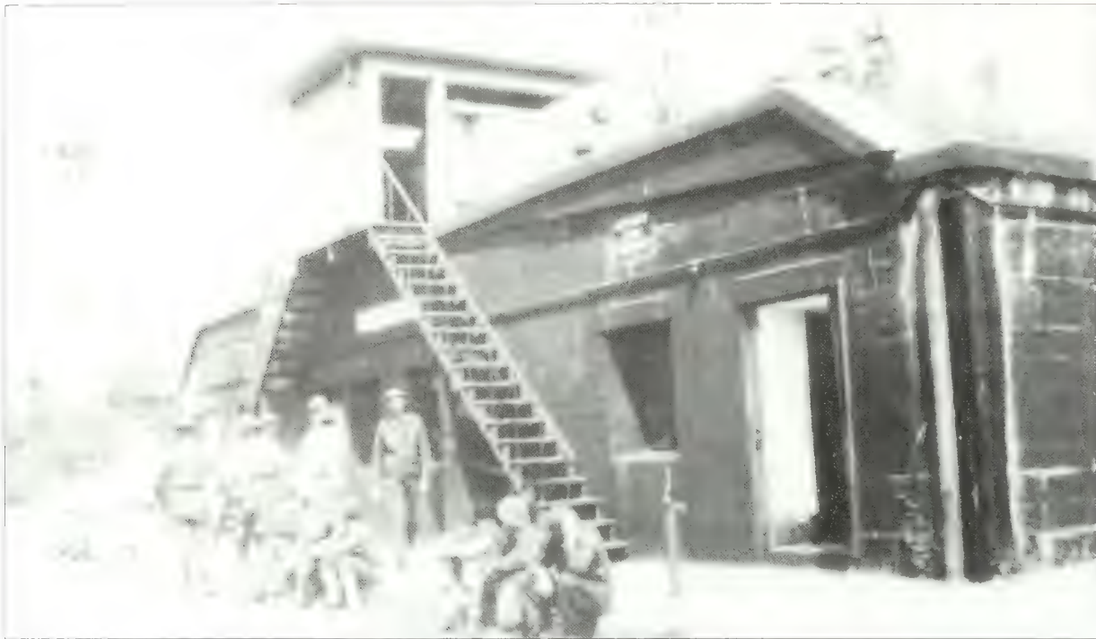
Figure 2.54. View looking northeast at Battery Gunnison, circa 1930-41. Although the east facade featured an engineered earthwork and planting compatible with the surrounding area, the west facade was not camouflaged or concealed. The concrete and metal framework of the structure was clearly visible when approaching from the west (Thomas Hoffman, Fort Hancock , Charleston, SC: Arcadia Publishing, 2007).
